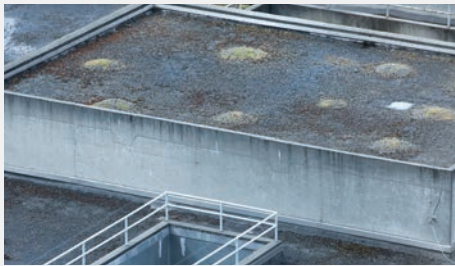
Waterproofing Roofs, Flat & Pitched
